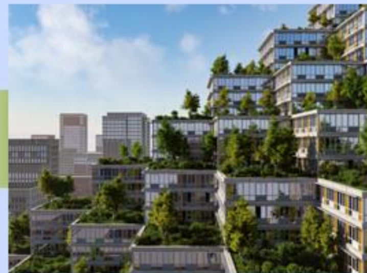
Irrigation of green roofs and green facades
